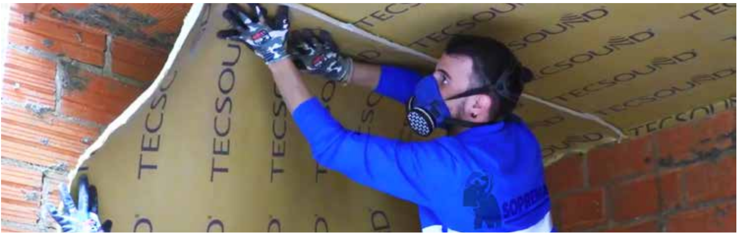
APPLICATION OF TECSOUND® FT IN FALSE CEILINGS
