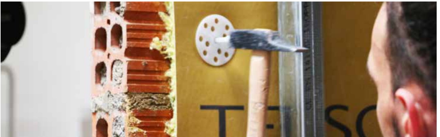
APPLICATIONS OF TECSOUND® FT WITH PTH FASTENERS
