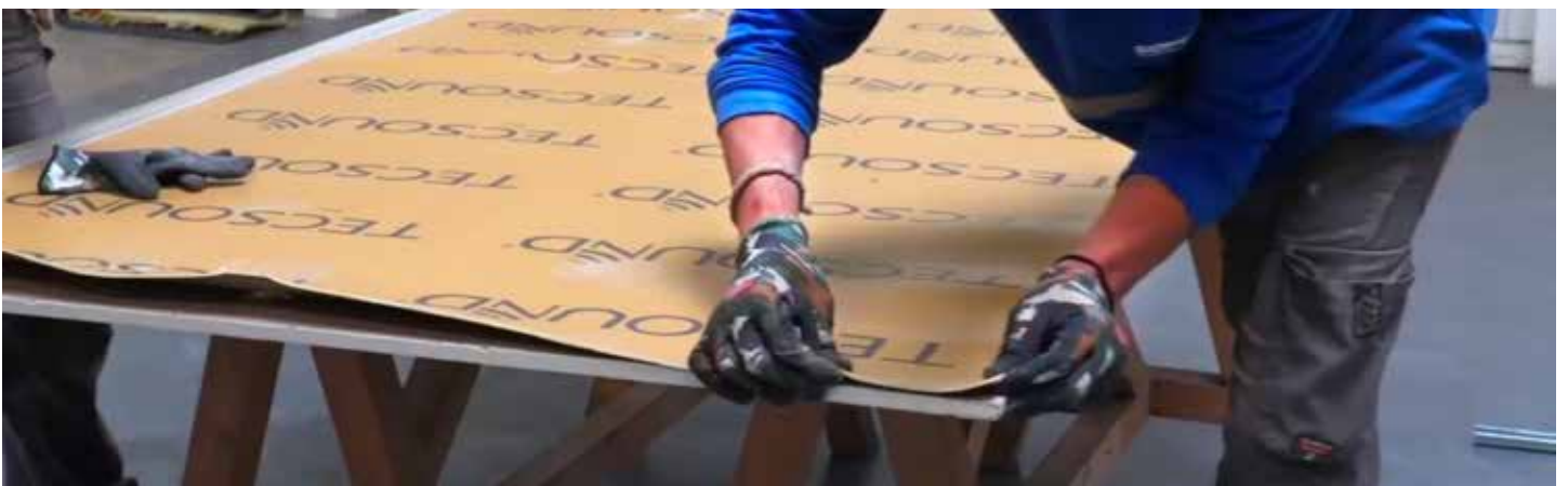
APPLICATION OF TECSOUND® SY IN DRYWALL PARTITIONS
